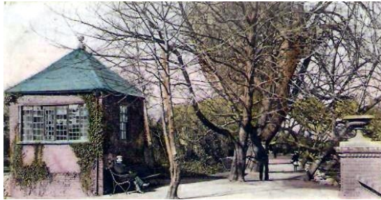
The demolished summerhouse by the riverside walk
