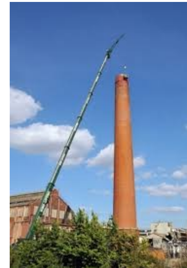
Demolishing the chimney stack
