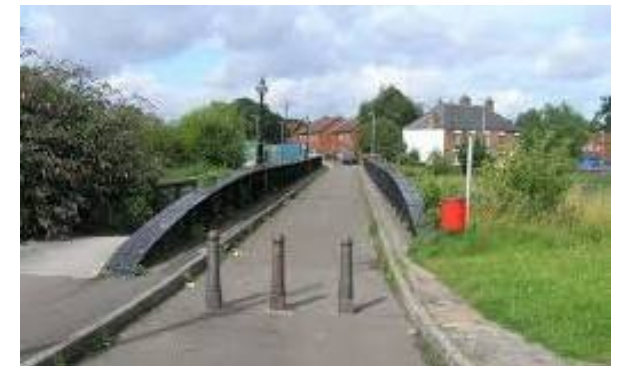
The pedestrianised telescopic bridge
