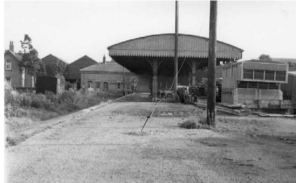
Bridgwater North station before demolition
