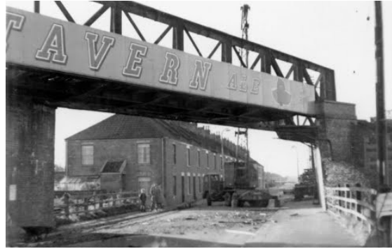
The demolition of the bridge over Bristol Road
